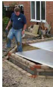
Insulation installed
