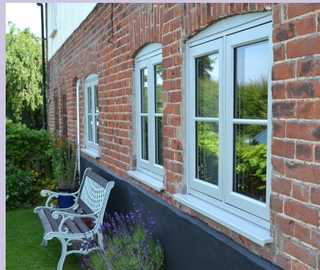
Flush Sashes, replicate timber design
